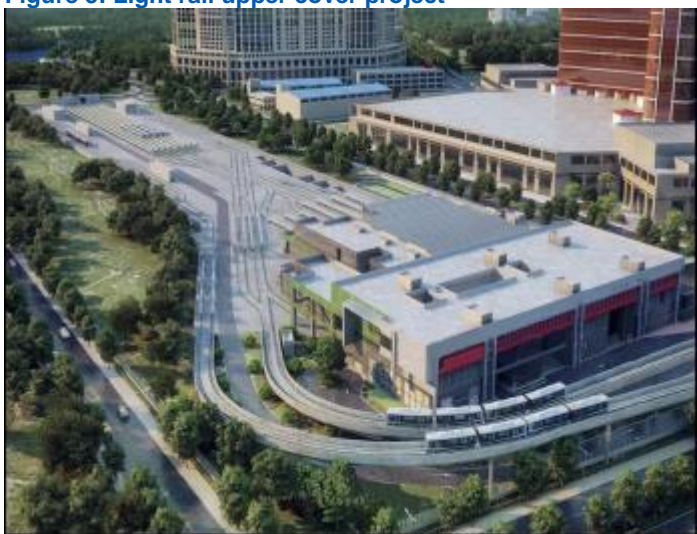
Figure 5: Light rail upper cover project
